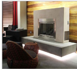
Toe Kick Lighting
